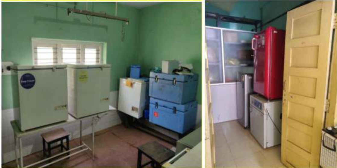
Equipment are kept on the tables and benches - Vandiperiyar CHC
