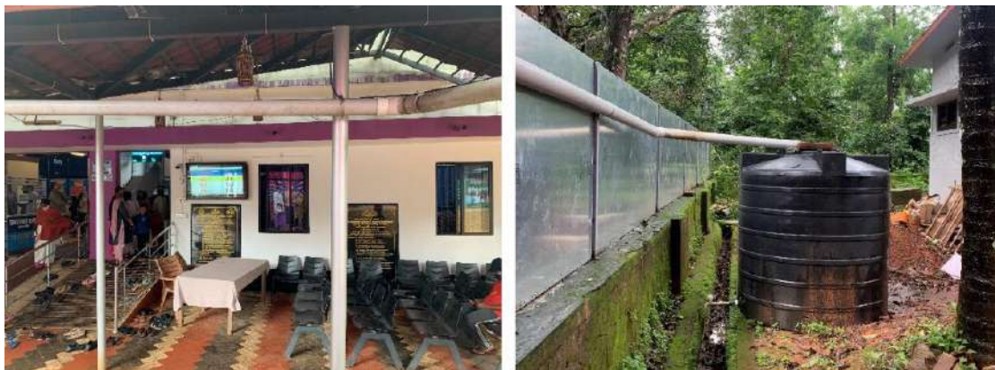
Rainwater harvesting setup at Noolpuzha FHC, Kerala
