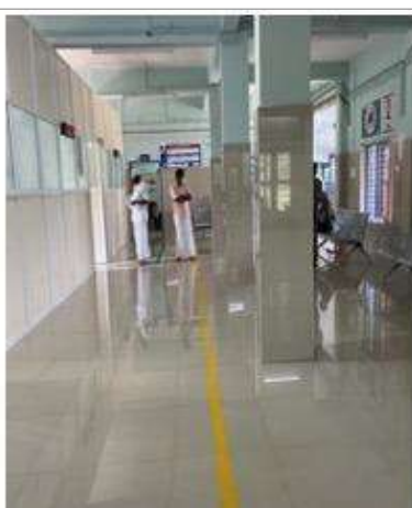
Newly constructed PHC floor with higher floor level, high wall tiling and ramps, FHC Pozhuthana, Wayanad, Kerala
